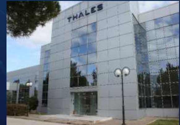
Country Office in Koropi, Greece
