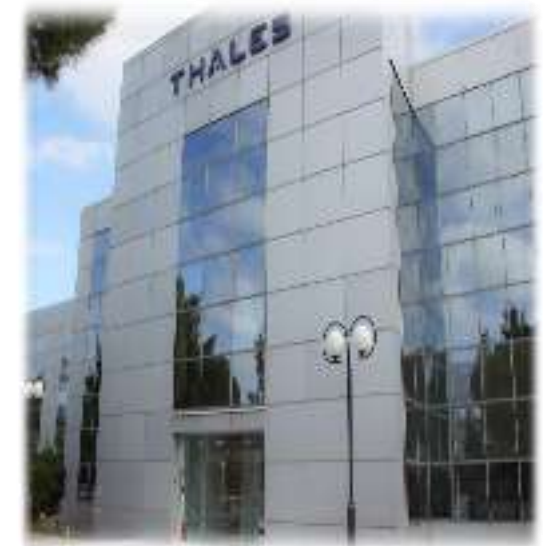
Country Office in Koropi, Greece
